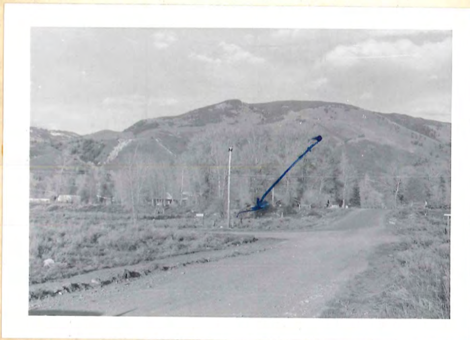
Looking Northeast over Lots A - I and K - Q; Block Eight (8) from a position west of intersection of Smuggler and Eighth Streets.
