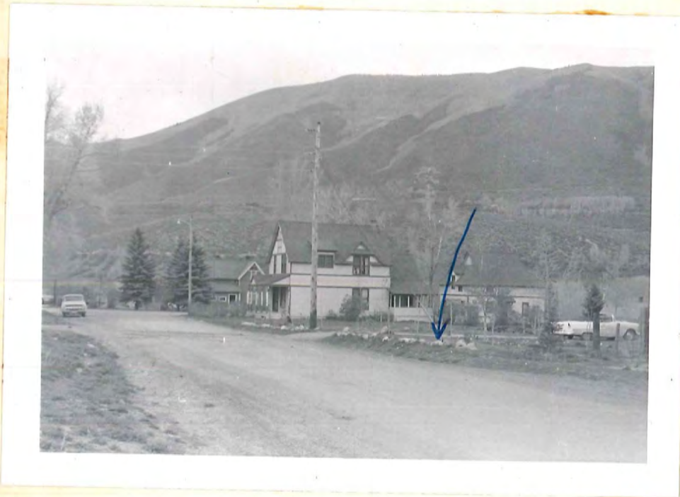
Looking north past Lot 4 and N 10' of Lot 5; Block 102 Hallam Addition from a position on North 3rd Street and South of subject.
